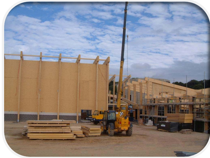
View of Hemsec Sips installed between glulam frames to Sports Hall.
