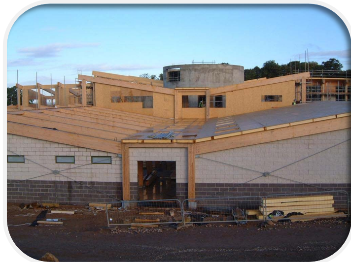
View of Hemsec SIPs roof being installed over the glulam frames.
