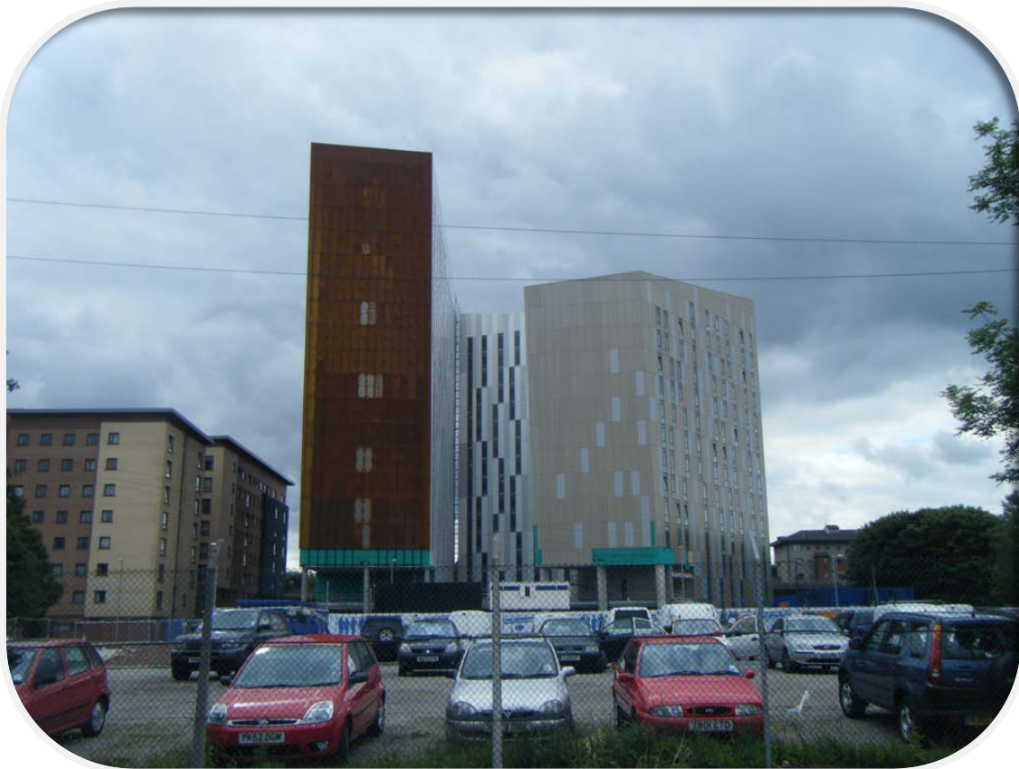
Finished with external cladding systems.
